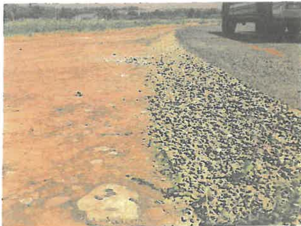
Compacted Base Rock
