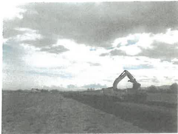
Stripping and Grading to Start Construction
