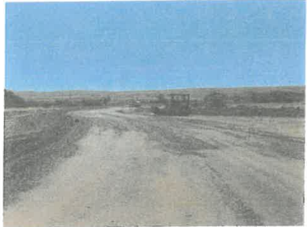
Water and Compact Sub-Grade and Base Rock
