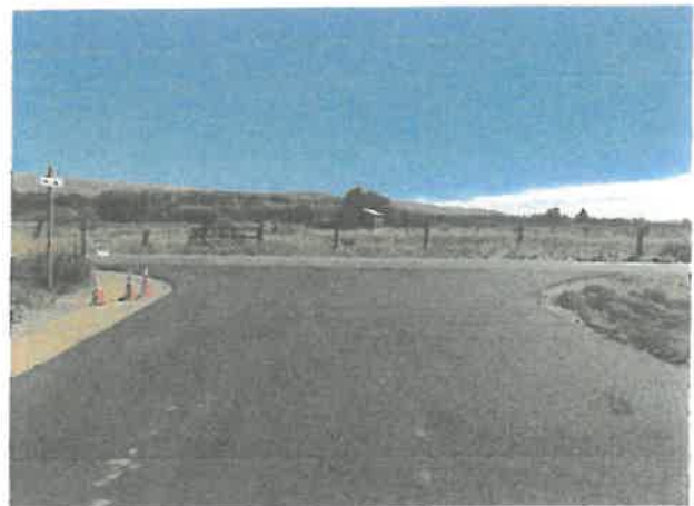
As-Built Paved Apron
